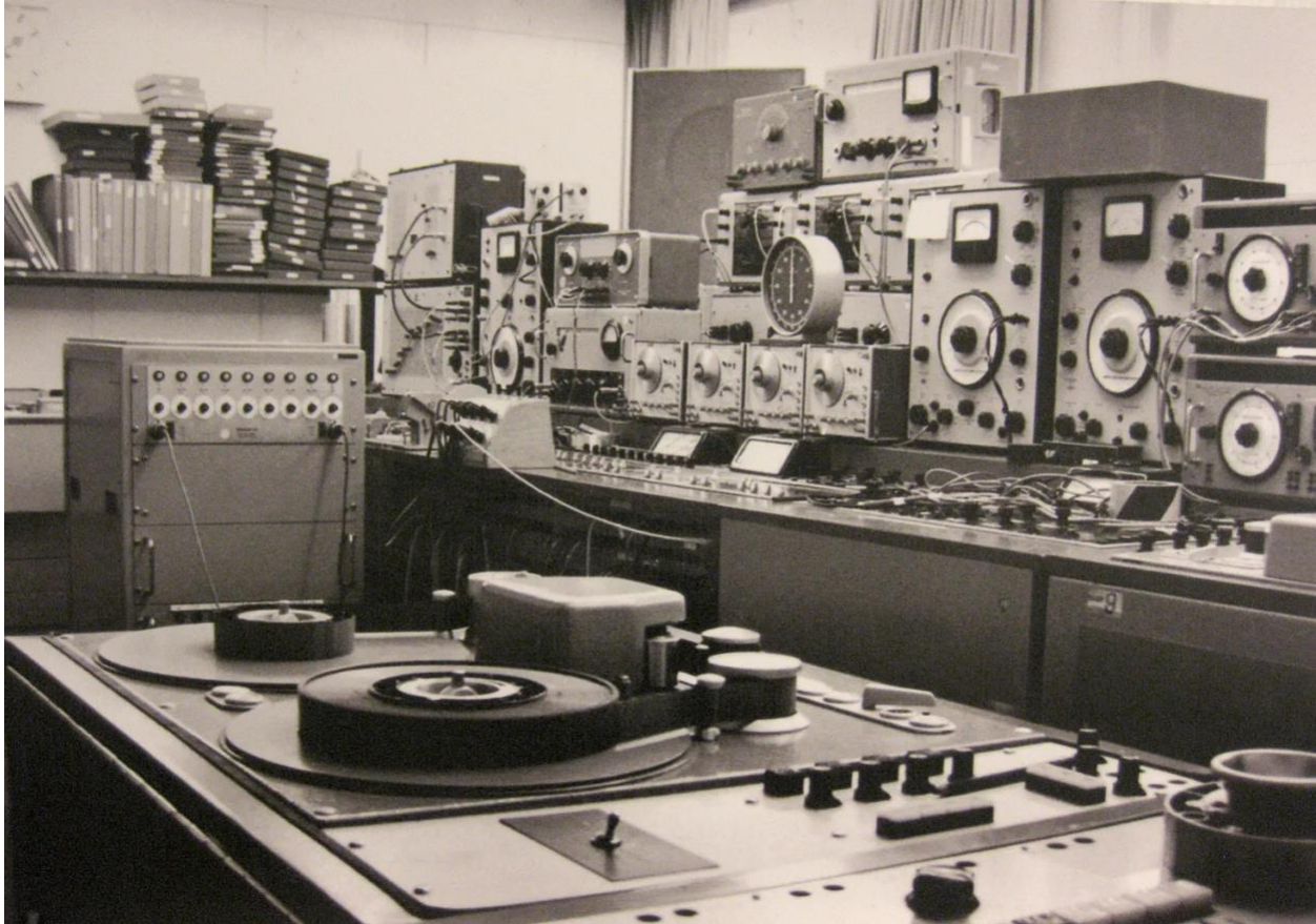
Figure 7.2 A four-track tape recorded and patched wave generators at the Westdeutscher Rundfunk studio. Date unknown (“WDR Electronic Music Studio, Werner Meyer-Eppler, Robert Beyer & Herbert Eimert, Germany, 1951”).
